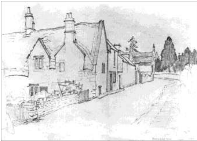
Fig.2 The ‘Thatched Cottages’ as they appeared in a sketch of 1939. Demolished despite their listed status.
