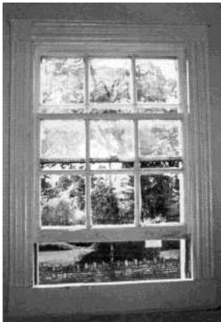
Fig.18 Window from a cottage built about 1820. Six-over-six panes within a reeded wood frame typical of the Regency period
