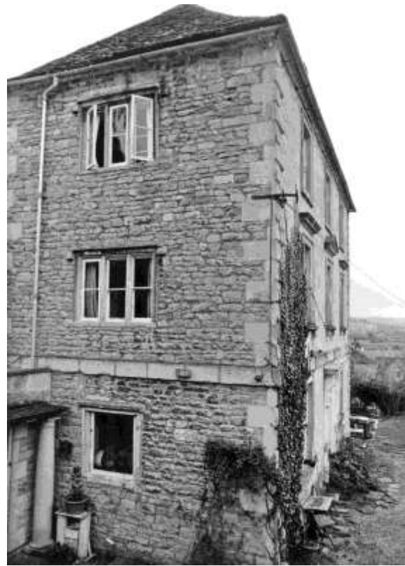
Fig.11 A classical mid 18th century façade on a late 17th century house
