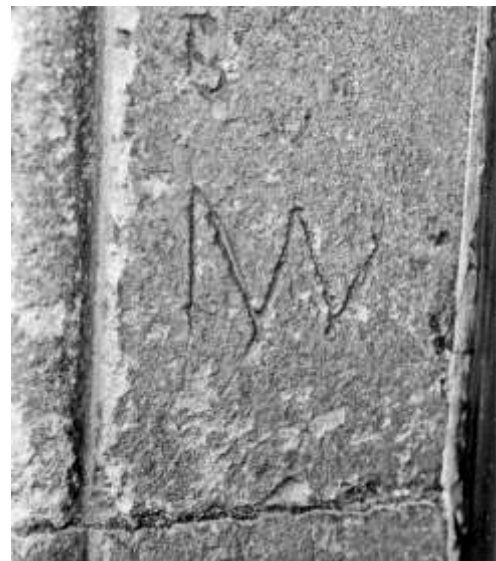
Fig.27 'M' (or 'W') on the door jamb of an early 17th century cottage.
