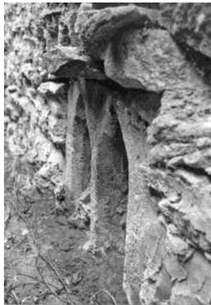
Fig.19 An unusual survival. A blocked medieval window in the rear wall of a house in the Batch, Batheaston. The house, which is not listed, has not yet been surveyed
